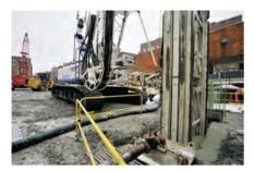
Located on Broadway between Quincy Street and Prescott Street in Cambridge, Massachusetts, the building will be a five-story addition to the original museum with two levels of below grade space. The foundation work consisted of the construction of SPTC (Soldier Piles Tremie Concrete) slurry wall that serves as a bulkhead to retain the surrounding soil for the site improvements during and after construction.
