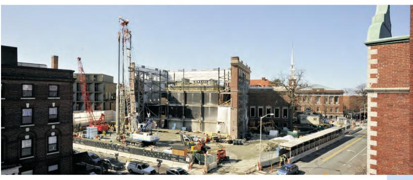
The 750 foot slurry wall was constructed as SPTC (Soldier Piles Tremie Concrete), with thickness of 36" and ran an average depth of 50 feet to accommodate the foundation layout and the particular design. More than 300 tons of steel and 3000 cubic yards of concrete were used in the construction of the SPTC Wall.
