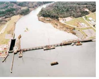
The Walter F. George Lock and Dam was constructed on the Chattahoochee River between 1955 and 1963 with the dual function of improving navigation and generating power. Its 82 ft. by 450 ft. lock can accommodate large barge traffic, while its four generating units with a plant capacity of 150 MW have an average energy output of 453,000 MWH.
