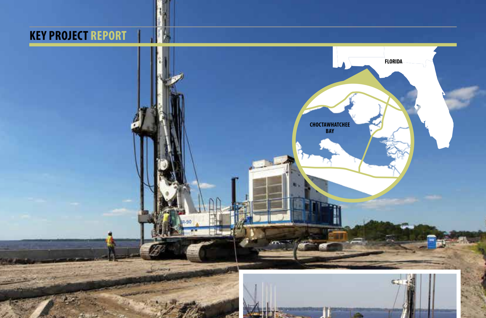
ABOVE: The Italian-built Soilmec rigs are handling a key portion of the US 331 widening project INSET: The link crosses the Choctawhatchee Bay in Florida RIGHT: The road is being widened so as to enable it to carry a greater volume of traffic
