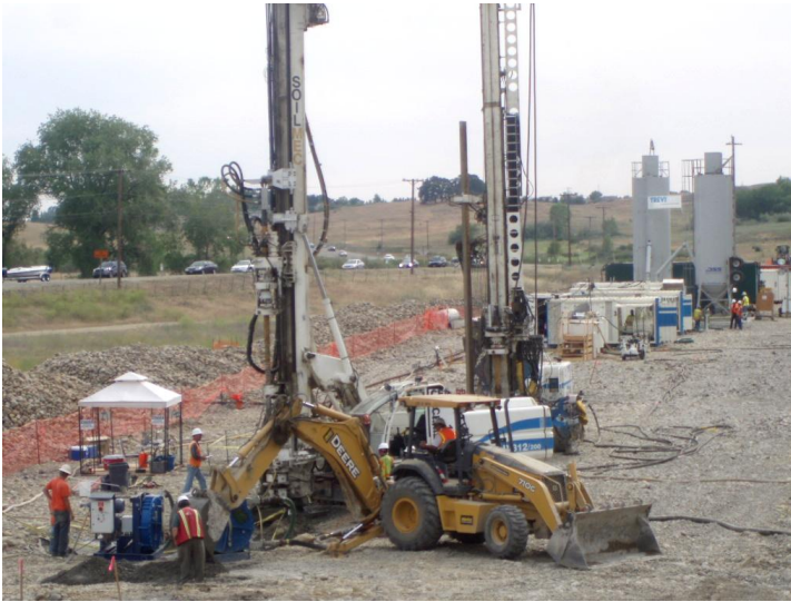
Pre-Drilling & Jet Grouting Operations
