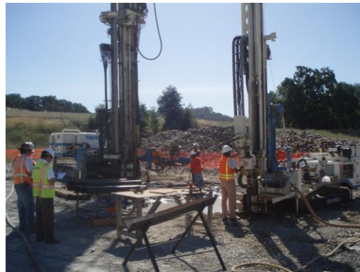
Pre-Drilling And Coring Operations
