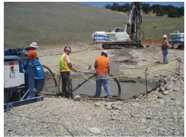
Spoil Management During Jetting
