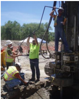
Verticality Checking
