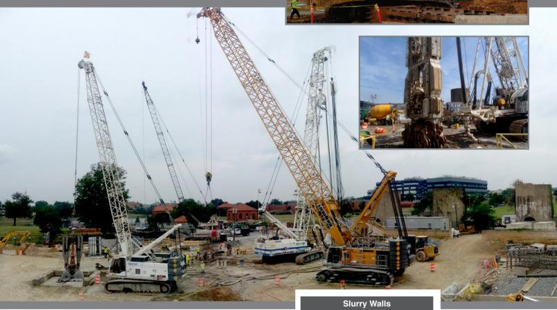
The slurry wall was constructed with various "soft eyes" where the tunnel boring machine was bored through to begin the tunnel excavation. GFRP bars were used in place of traditional black steel at pre-determined locations to accommodate slurry wall opening requirements for the tunnel boring machine.
